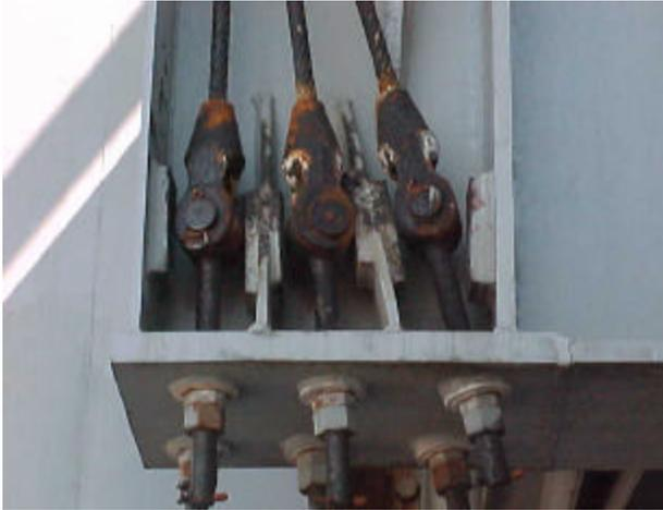
Typical corrosion on the Deck Edge Elevator cables
